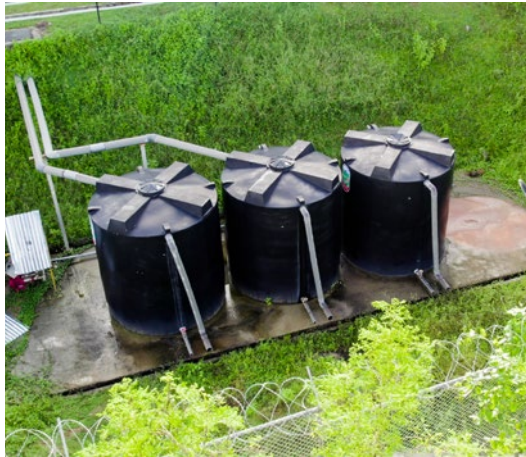
Rainwater harvesting with 4,752m 3 capacity tanks at the Pharmaceutical Manufacturing Facility in Homagama where the collected water is used for gardening
